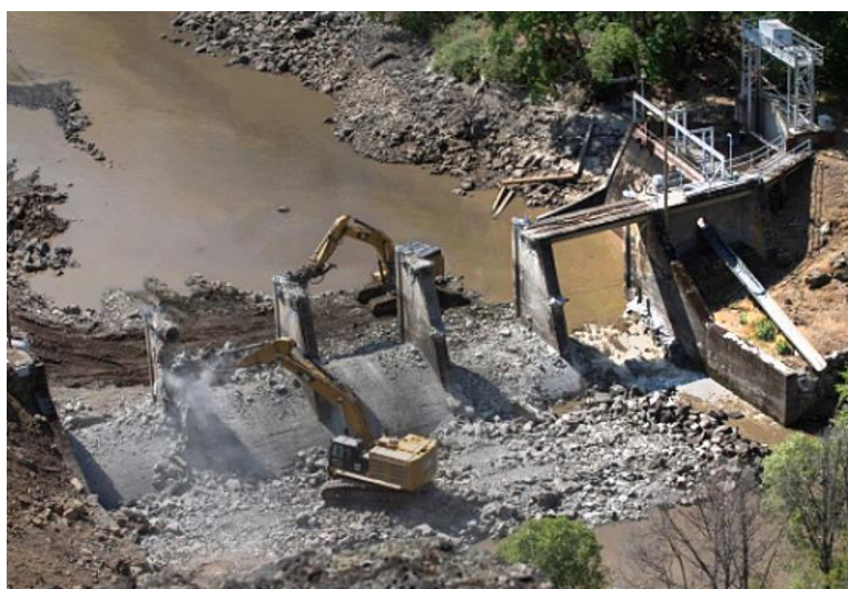
Copco Dam 2 removal was completed in July 2023.
